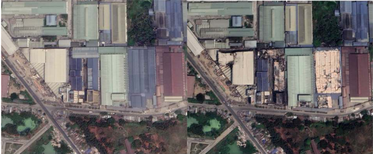
Figure 48: Satellite imagery of visibly fire damaged factories corresponding to SM0243.
