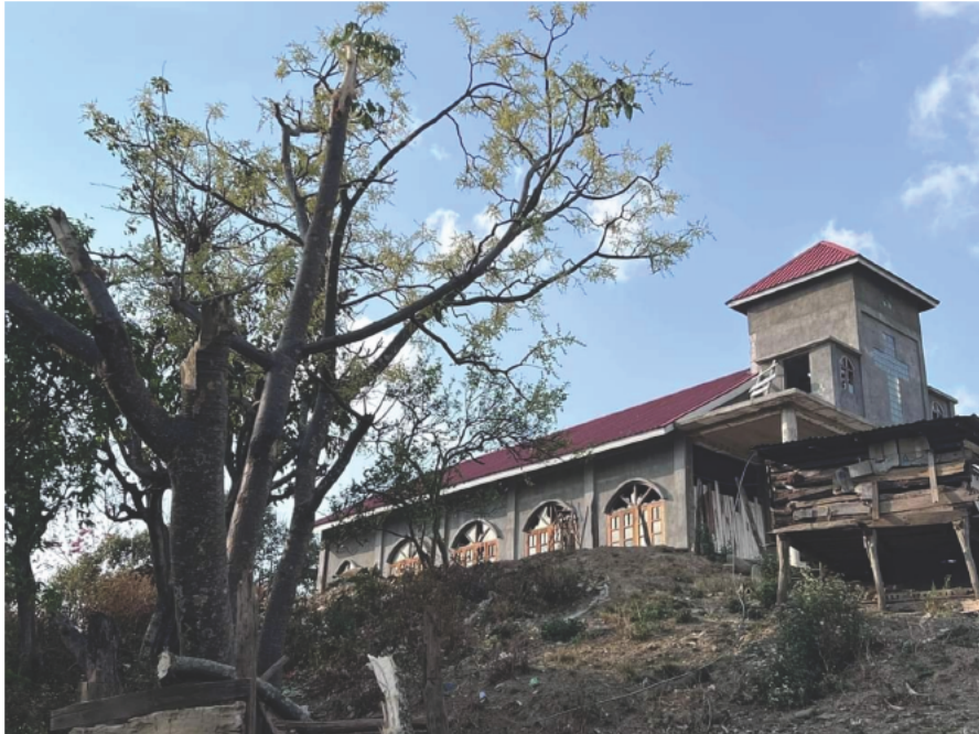
Figure 8: It is alleged that Kuafo Baptist Church was damaged following airstrikes on 30 March. UGC shared on the day appears to show smashed windows [22.751632, 93.425222] (source: Khonumthung Burmese , warning: graphic link).
