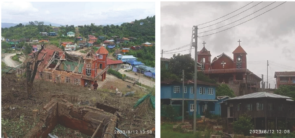
Figure 27: Timestamped UGC shows extensive structural damage to Ramthlo Baptist Church (sources: Burma Media Consortium ; The Chin Journal , warning: graphic link).
