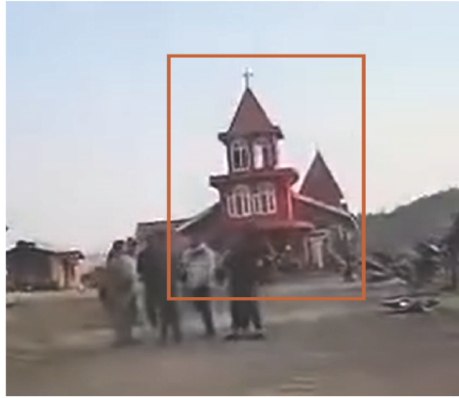
Figure 18: Tlanglo Baptist Church (shown here in the brown box) is visible in UGC shared on the day of the alleged airstrike. Owing to the low resolution of this footage, Myanmar Witness was unable to verify damage to the church building [23.008091, 93.336918] (source: Global Tlanglo Youth Organization - GTYO ).
