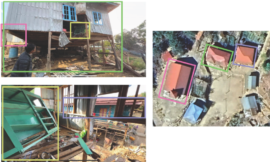
Figure 9: Myanmar Witness has geolocated footage showing significant damage to the residential buildings which neighbour Khuafu Baptist Church, shown here in the pink box [22.752130, 93.425063] (source: Ayeeyarwaddy Times , warning: graphic link).
