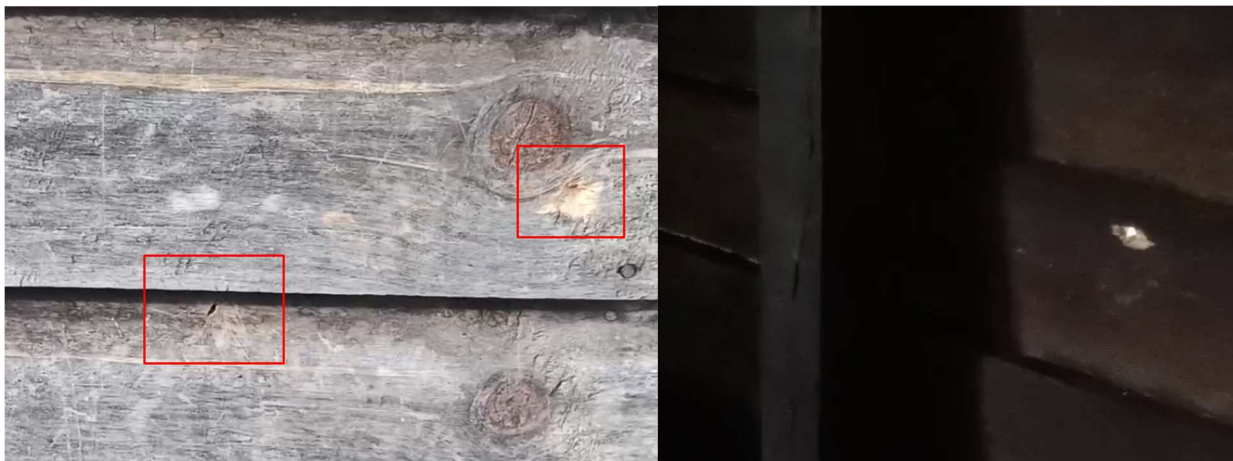
Figure 12: Two marks on the child's home, one having penetrated fully (left) and another with no entry penetration (right). The hole shows a small penetration entrance and a larger penetration exit with more splintering and fresh wood, with the rightmost pieces of damage exposing fresh wood on the wall, penetrating it but with no exit penetration on the side of the wall. This could indicate a fairly recent penetration with force into the wood to cause this kind of splintering, as well as multiple markings.
