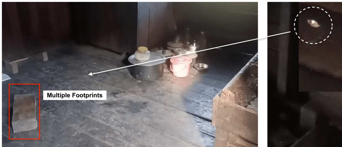
Figure 14: Images of the inside of the home, where multiple footprints can be observed which could suggest there was recent activity in the home. The arrow here represents that the hole in the wall potentially aligns with the stool in the image (red box) - where the child could have been seated at the time of this incident - especially if the child was, as reported, eating at this time.
