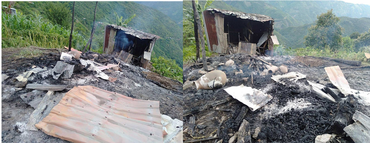
Figure 23: A structure appears to have been destroyed in Kyam Ain Nu (ကြာအိမ်နူး) village, there appears to have been a structure destroyed initially and another structure that was part of the original is still standing - likely a toilet or shed.
