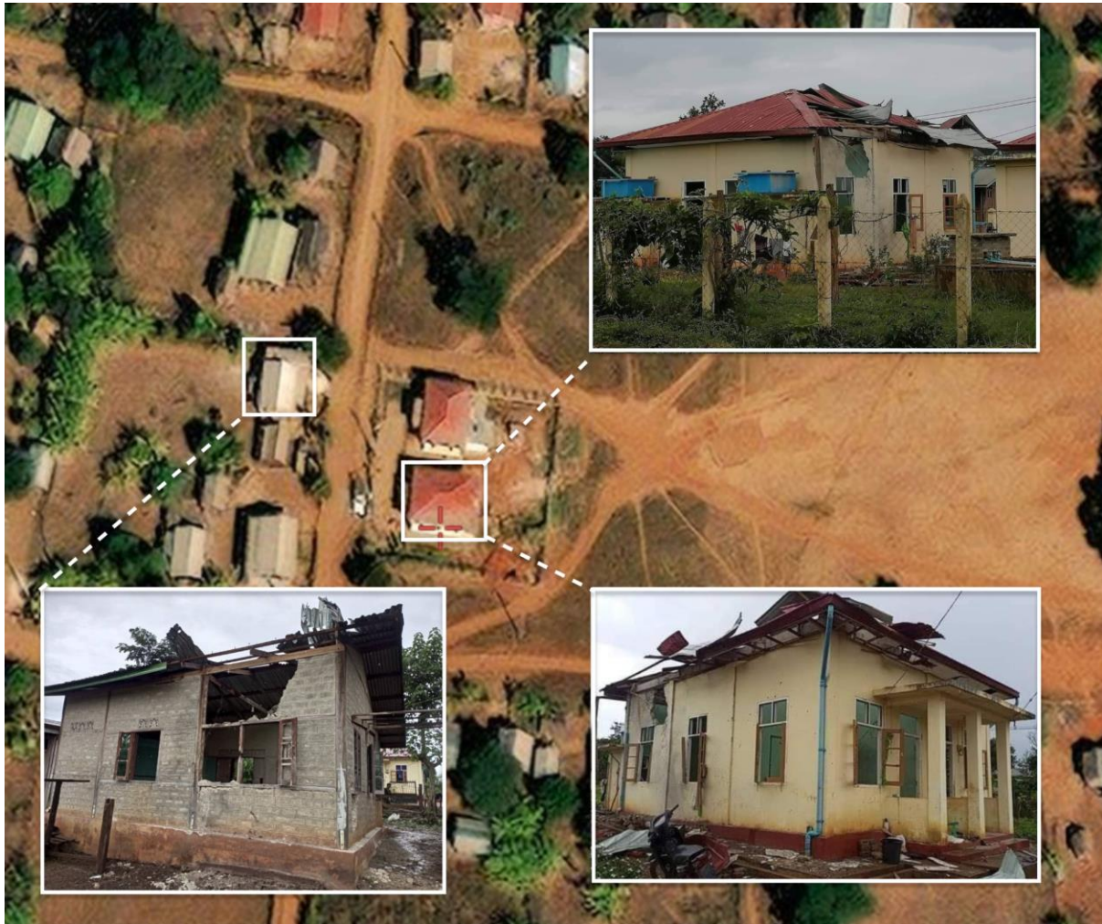
Figure 24: Geolocation image of Daw Parpa village, highlighting the destroyed clinic area - with red roofing - and residential buildings (source: private).
