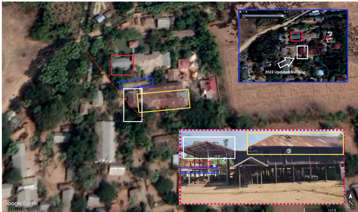
Figure 30: Geolocation of a damaged school building in Let Yet Kone village.
