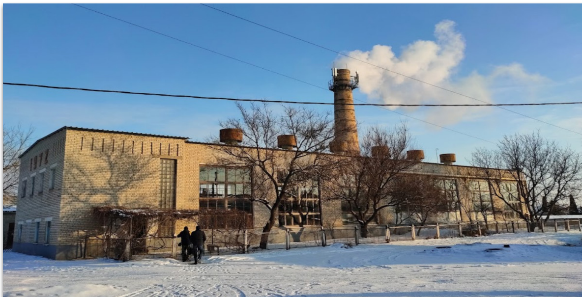
Figure 27: Google Maps imagery of the municipal boiler plant, including distinctive chimney stack. 52
