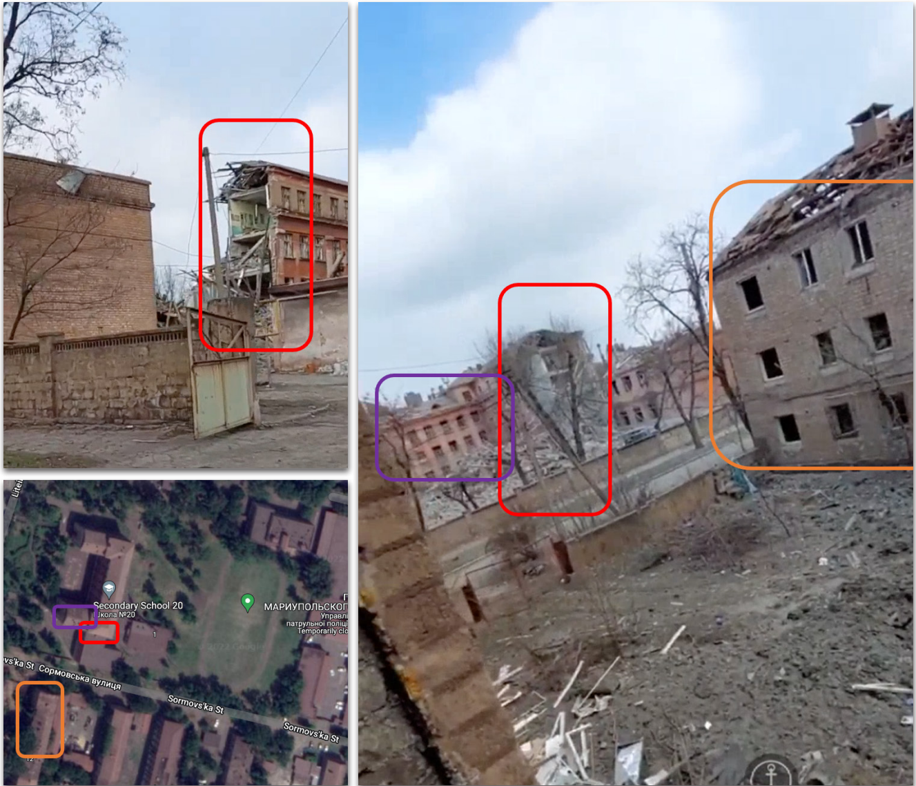
Figure 14: Partially destroyed school N°20 in Mariupol, Donetsk oblast [47.136495, 37.578732].
