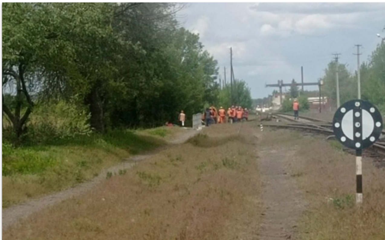
Figure 3: Railway repairs outside 'Starobilsky Elevator LLC'. [Image taken from 49.282288, 38.927680, facing North]. 14
