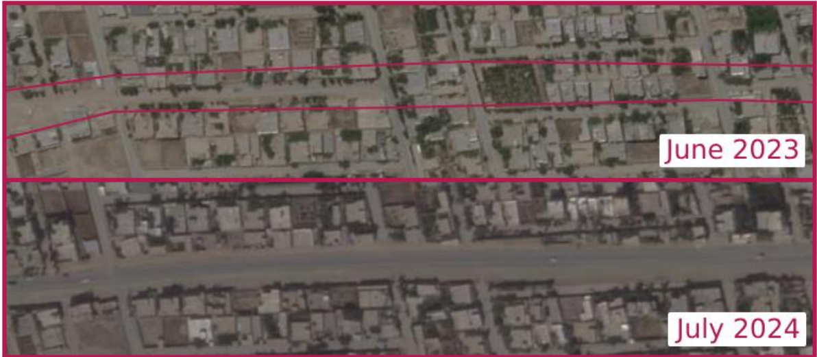
Figure 19: Satellite images from Planet showing the before and after demolitions of residential properties in PD 17 [34.574711, 69.079603]. Image © 2023 & 2024 Planet Labs Inc. All Rights Reserved. Reprinted with permission.
