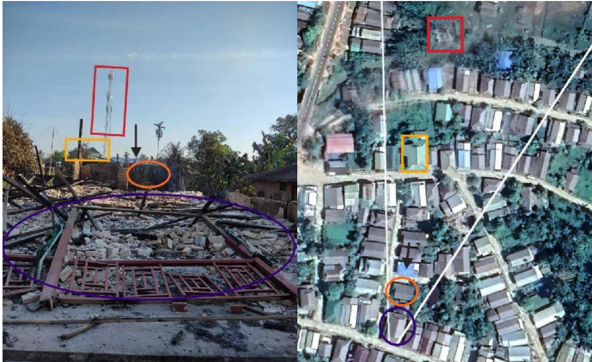
Figure 6: Geolocation of damaged houses in To village [12.865856, 98.660519] (Source - The Tanintharyi Times ).
